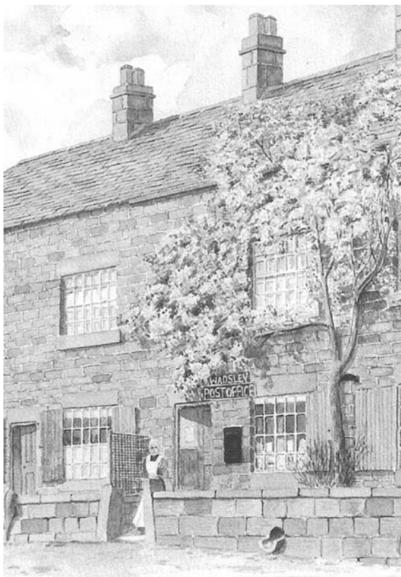
Figure 1 – Wadsley Post Office in the 19 th Century. Reproduced with permission of the artist C.P. Kaye.
